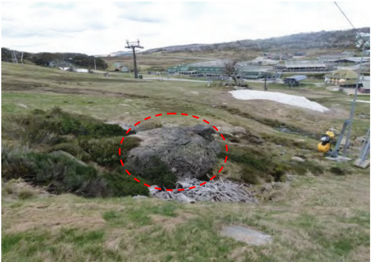
Photo 6: This rock at the bottom of the Slopestyle course will be blasted with rock fragments placed in the depression surrounding the rock.
